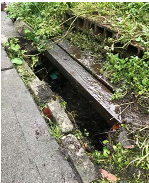
Figure 4 – Alley Springs in the 'sand box' drainage structure
